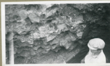
10. H.2-4. from N Rubble fill (mixed -in-situ water worn boulders) behind ashlar face (remnant beyond head of figure.)
