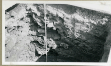
9. 93 East North Drawbridge pier 1st end abutting on solid rock. Rubble fill L. Solid R.
