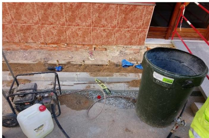
Sectional pressure test and disinfection of water pipes PE 150. For disinfection  $\text{NaClO}_2$  was used.
