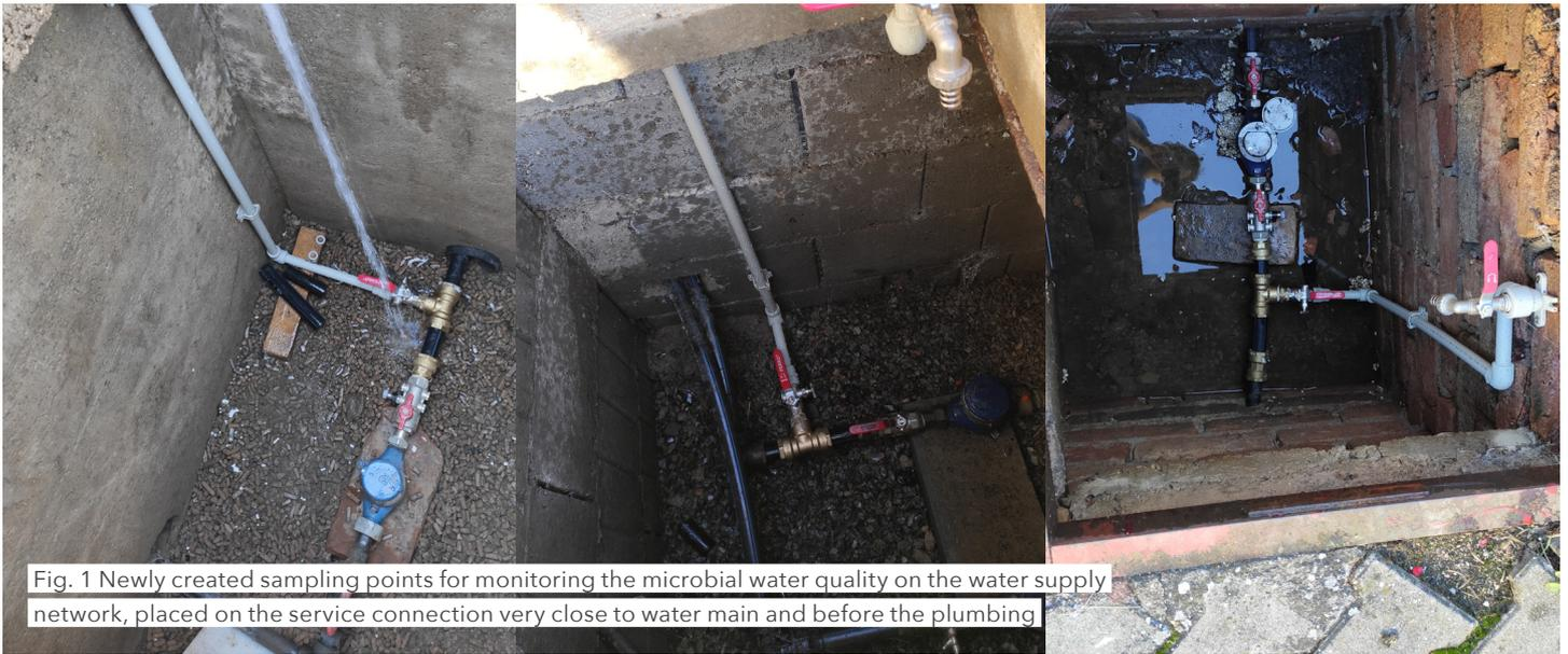
Fig. 1 Newly created sampling points for monitoring the microbial water quality on the water supply network, placed on the service connection very close to water main and before the plumbing
